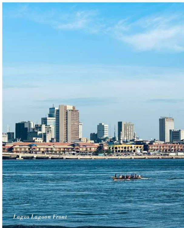
Lekki-Ikoyi Link Bridge
